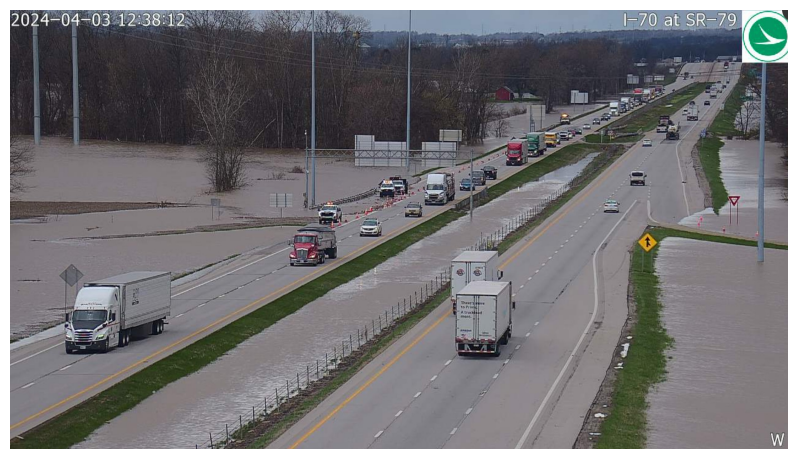
Figure 8: Photo taken from Ohio Department of Transportation street camera on I-70 as water overtakes highway on April 3 rd , 2024. Courtesy of Ohio Department of Transportation ( https://www.transportation.ohio.gov/ ).
